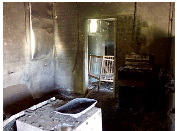
6. Interior of structure: kitchen.
