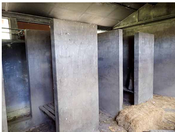
7. Interior of structure: showers.
